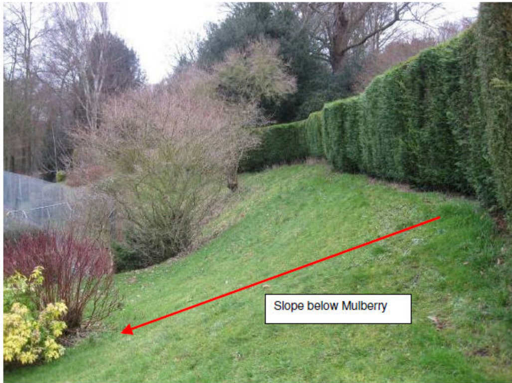
View of slope below extension to Mulberry from South
