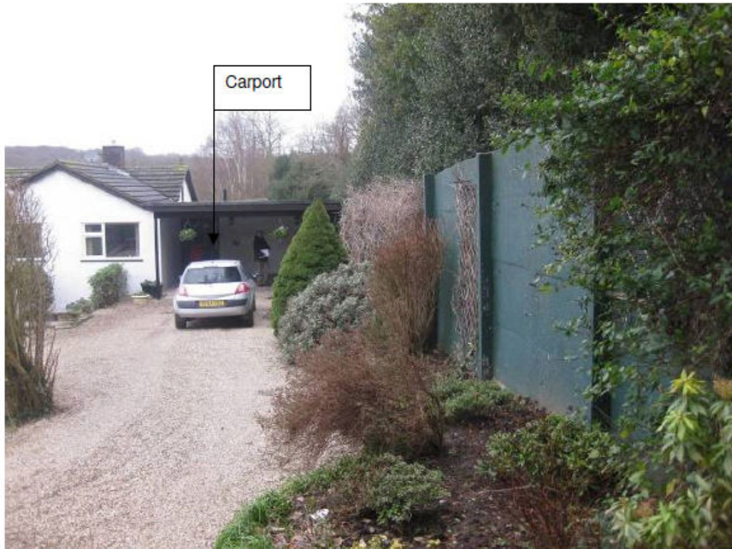
View of Mulberry from South Showing Boundary Wall to Dryads Hall and Carport
